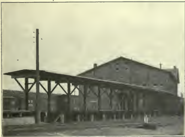
FIG. 319. FREIGHT HOUSES. Freight Transfer Station of the Chicago & North Western Railway at 14th Place and Oakley Avenue, Chicago.
